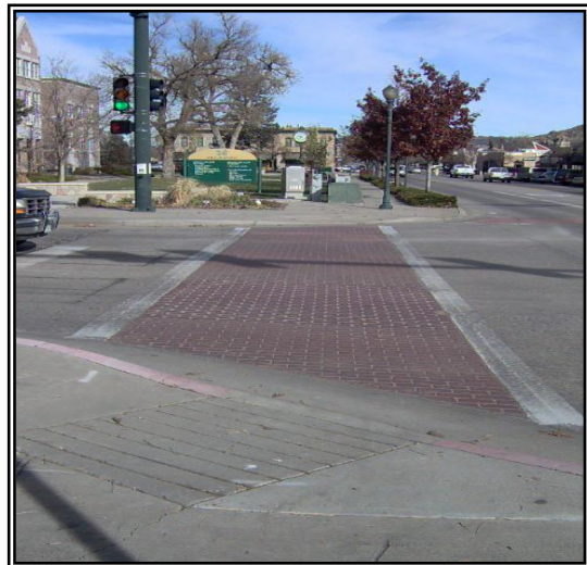
Brick pavers are utilized to provide a visual and textural delineation at this traffic intersection.
