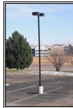
The use of down-shielded fixtures is to prevent light glare and light trespass.
