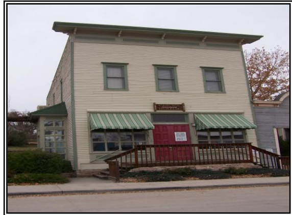
Carlson Building: Well-defined building base, middle, and top (cornice); high-profile entry with transom window; orientation to street, and complementary awnings, make this a simple but classic western building.
