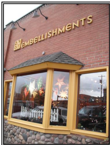
Choice of window type and window treatment can make or break a building.
