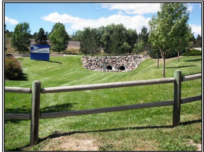
Supplementing natural drainage areas with appropriate trees, shrubs, and grass makes an attractive stormwater feature and as part of a site landscape plan.
