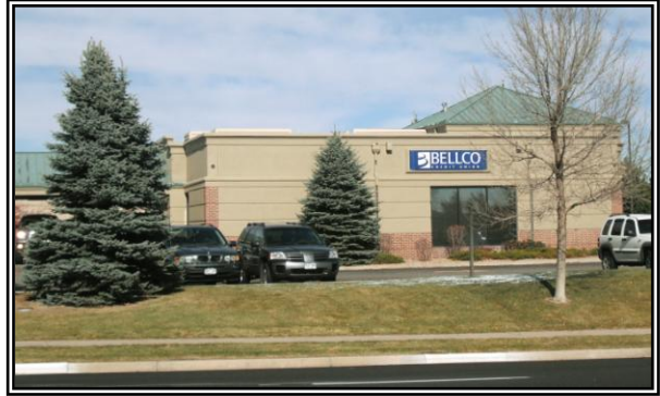
Rooftop mechanical equipment screened with compatible material.
